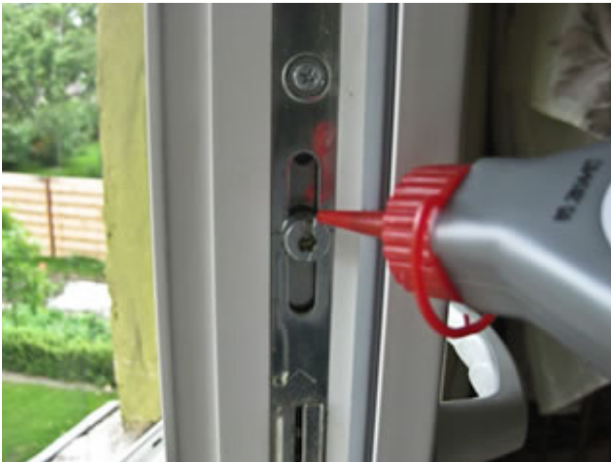
Lubricating window, door hardware.
